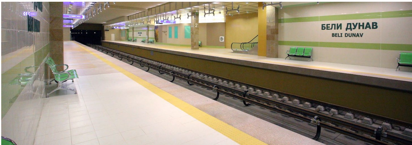
BELI DUNAV METRO STATION Sofia, Bulgaria
